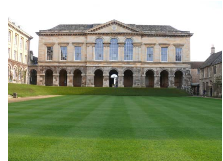
Main Quad looking East towards the Main Block
