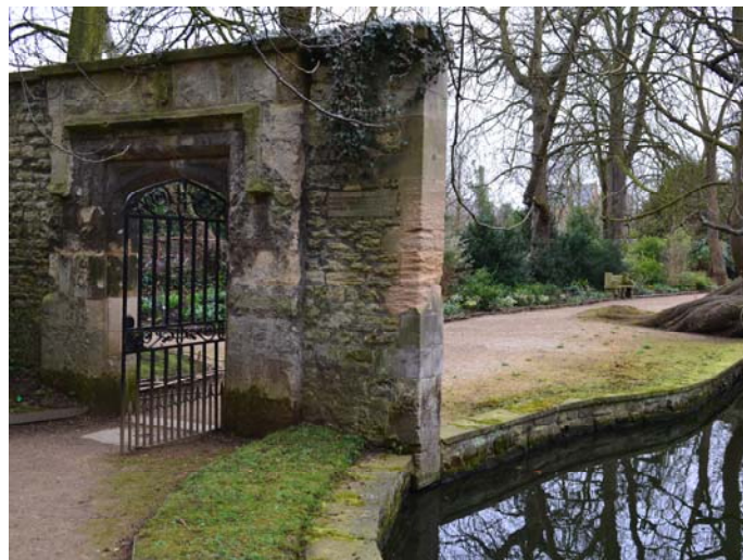
Listed feature gate & archway adjacent to the lake
