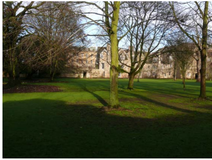
Looking NNW from the Linbury to the Medieval Building
